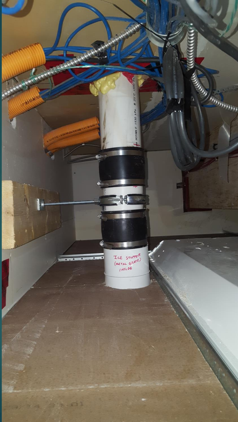
Inside drop ceiling
